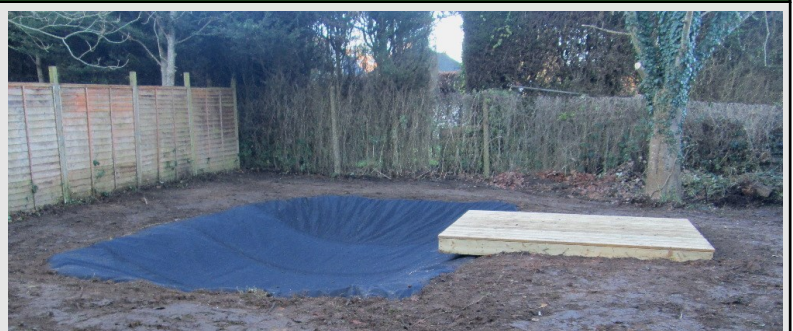
The wildlife pond under construction, showing the butyl liner
